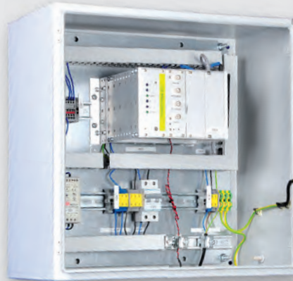
The test system was implemented as a complete system in a wall-mounted enclosure – with integrated ICP amplifier and NI Single-Board RIO.
